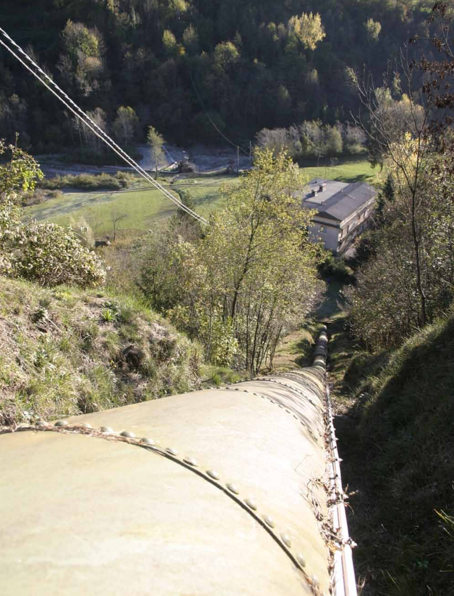
Power plant at Piazza
